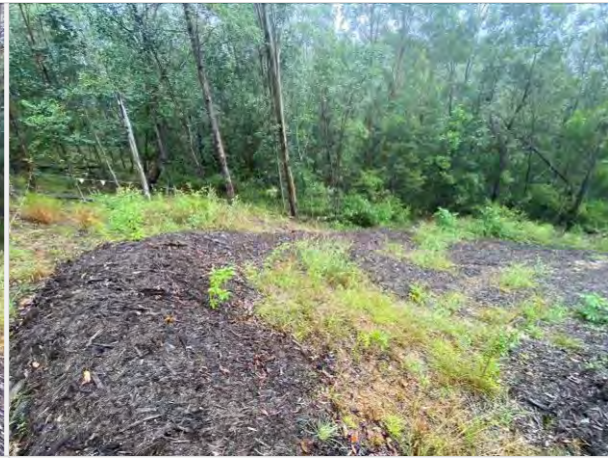
CLEARING PHASE IMAGE RETAINED HABITAT BEHIND VEGETATION PROTECTION FENCING AND MULCH BERM
