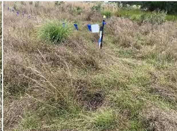
Protection Fencing Requiring Repairs
