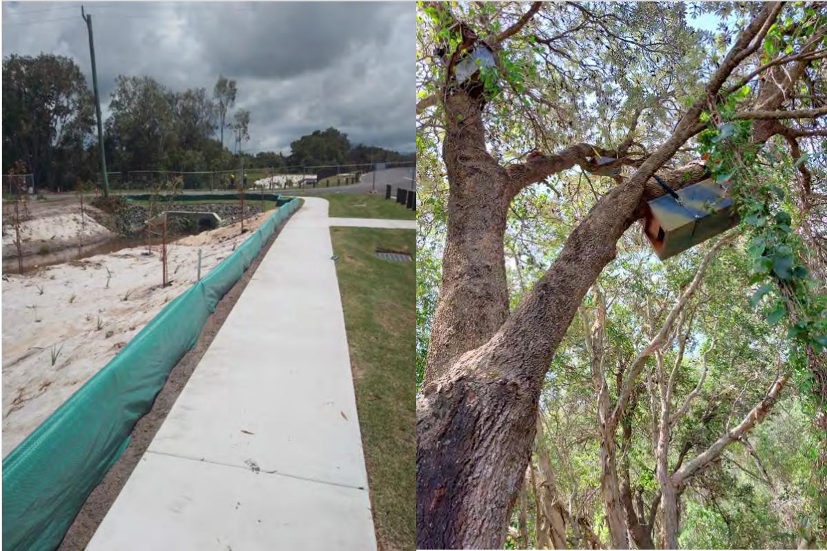
Frog Fencing Installed Between Frog Habitat Zones
