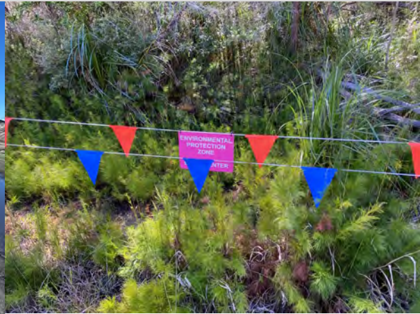
Tree Protection Fencing and Signages Installed Externally to the Retained Frog Habitat Zone
