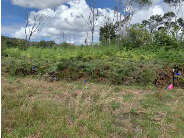
INCIDENCE OF NON-COMPLIANCE TO BE RECTIFIED: FENCNG REQUIRING REPAIRS
